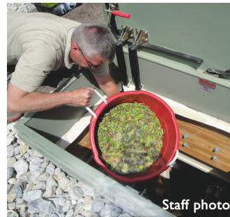
Jeff Jabco lifts up a bucket of sedum clippings to be planted on the roof
