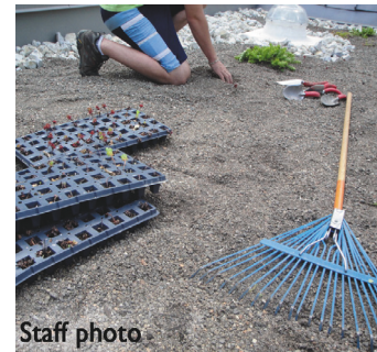
Planting sedums on the Wister roof
