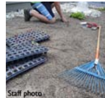
Planting sedums on the Wister roof
