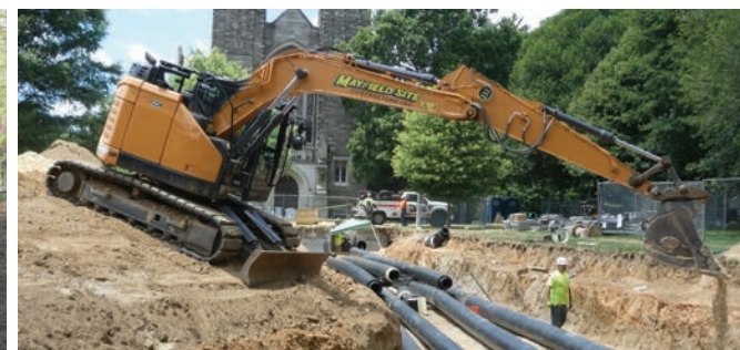
Laying infrastructure piping in Parrish Lawn as part of the College's Zero by 35 initiative.
